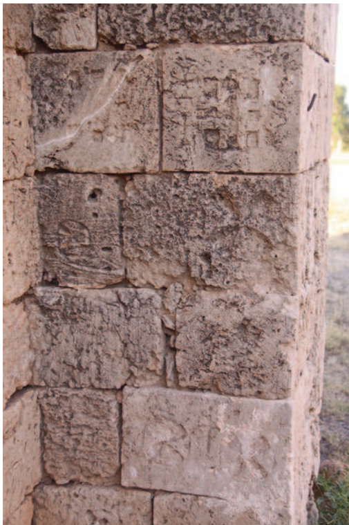
Fig. 5.5 Crosses carved on the eastern buttress, southern facade, ©Photograph by Michele Bacci
