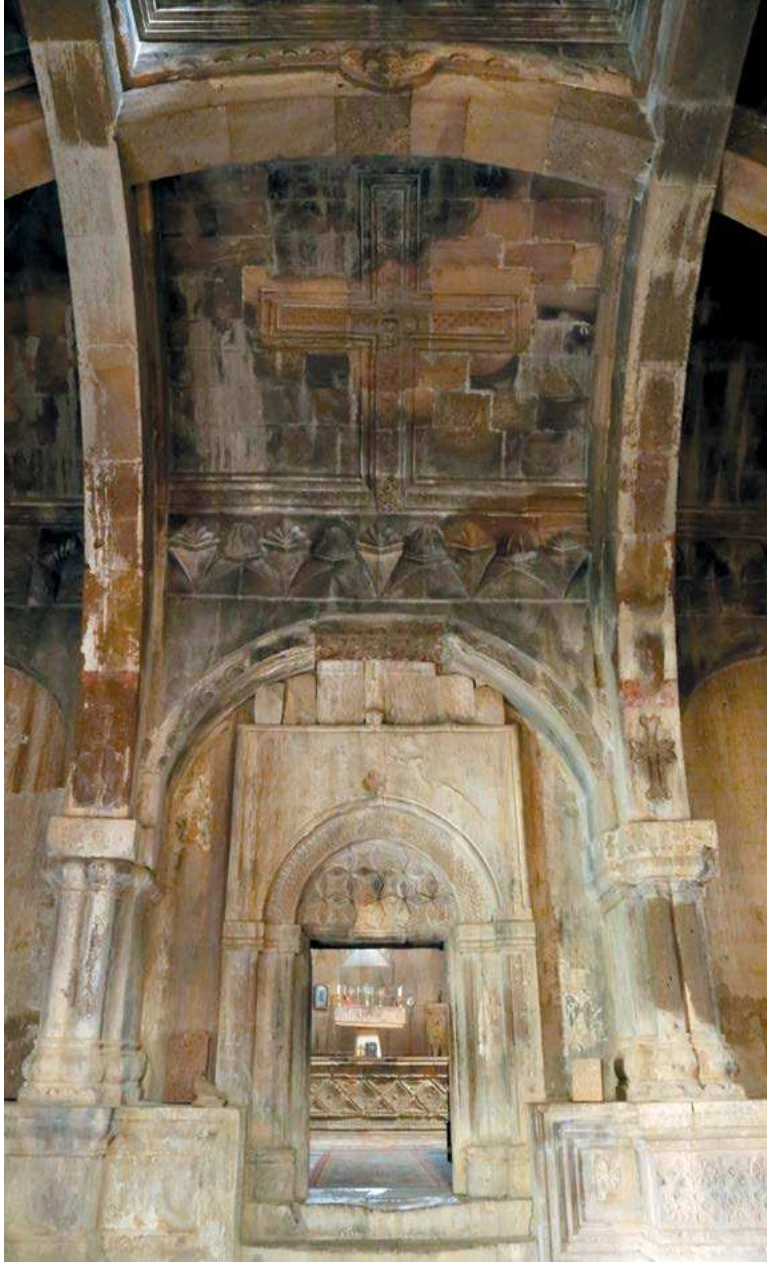
[17] Doorway between gawit 45 and church (1240), Gandzasar
