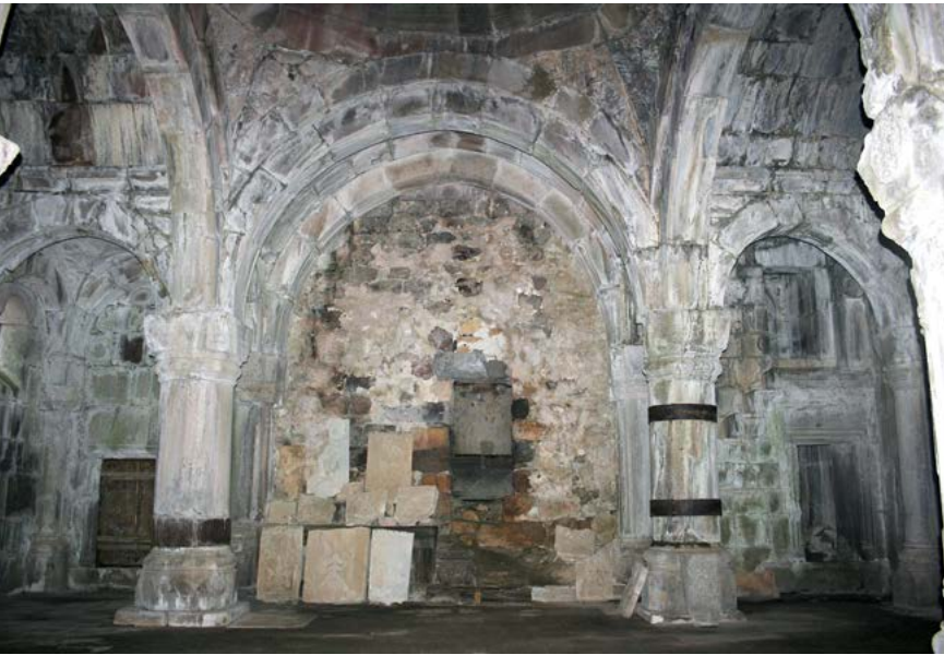
[6] Doorway between gawit 6 (before 1224) and the old church, Makaravank 6
