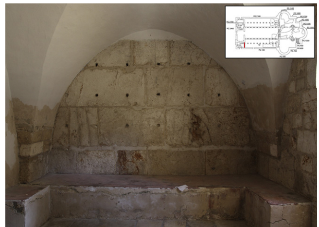
Fig. 36. Elevation 3300. System of cavities which served to anchor the marble slabs.
