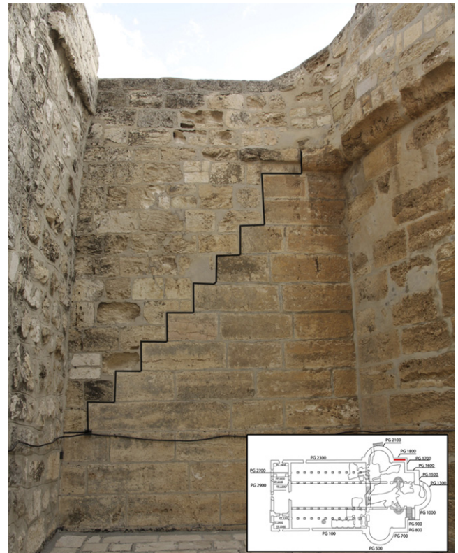
Fig. 23. Elevation 1800. The line shows the reconstructed section of wall.
