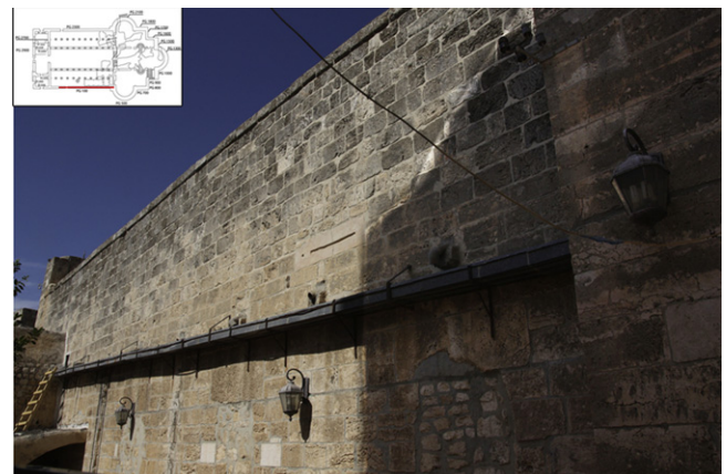
Fig. 8. Exterior wall of south aisle, with blocked up windows.
